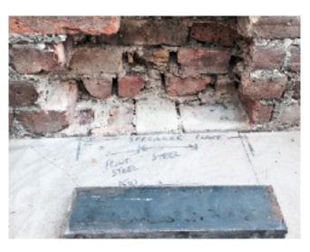
The mortar is carefully drilled out on our side and the bricks are removed without disturbing the neighbouring property. The wall is 225 mm thick and as our steel bearer plate only needs 100 mm of bearing there is no chance of damage to the other side.
