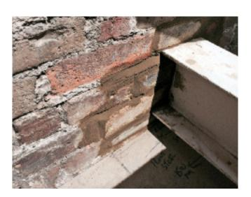
Once the steel is levelled and in position the hole is bricked back in and made good.
