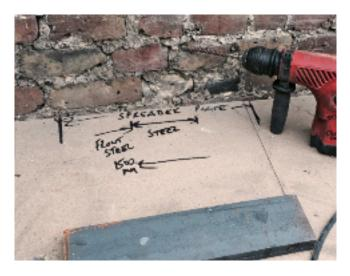
The steel beam and the bearer plate location are marked out as shown.
