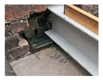
The bearer plate is then bedded on a cement base, levelled and allowed to set. The following day the steel is positioned centrally on the bearer plate. Our steel beams are fabricated in sections with a bolted splice joint to avoid the need to cut completely through the wall to get them in position.
